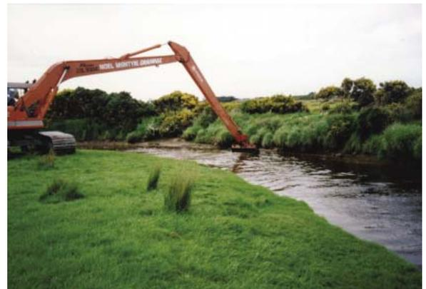
Channel excavation work carried out from the side where the least disturbance will be caused.
