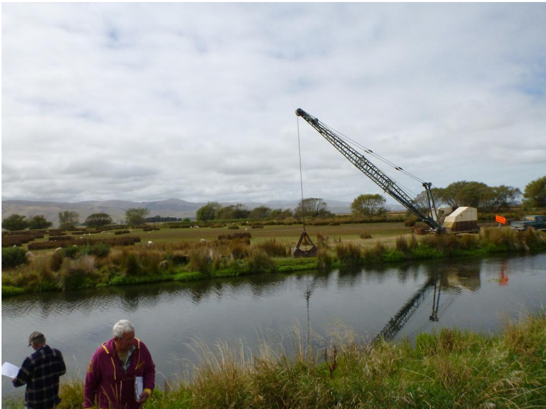
Photo shows the crane removing weed from the stream
